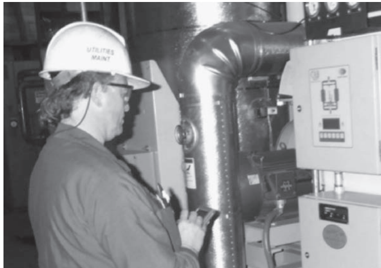
FIGURE 5.6. Tradesman collecting readings using the reliability software on a pocket PC, with instantaneous feedback on alarm conditions. (Courtesy of Ivira Corporation.)
